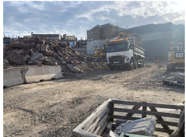
Material being removed from site
