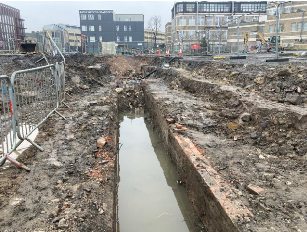
Service tunnel to be broken out
