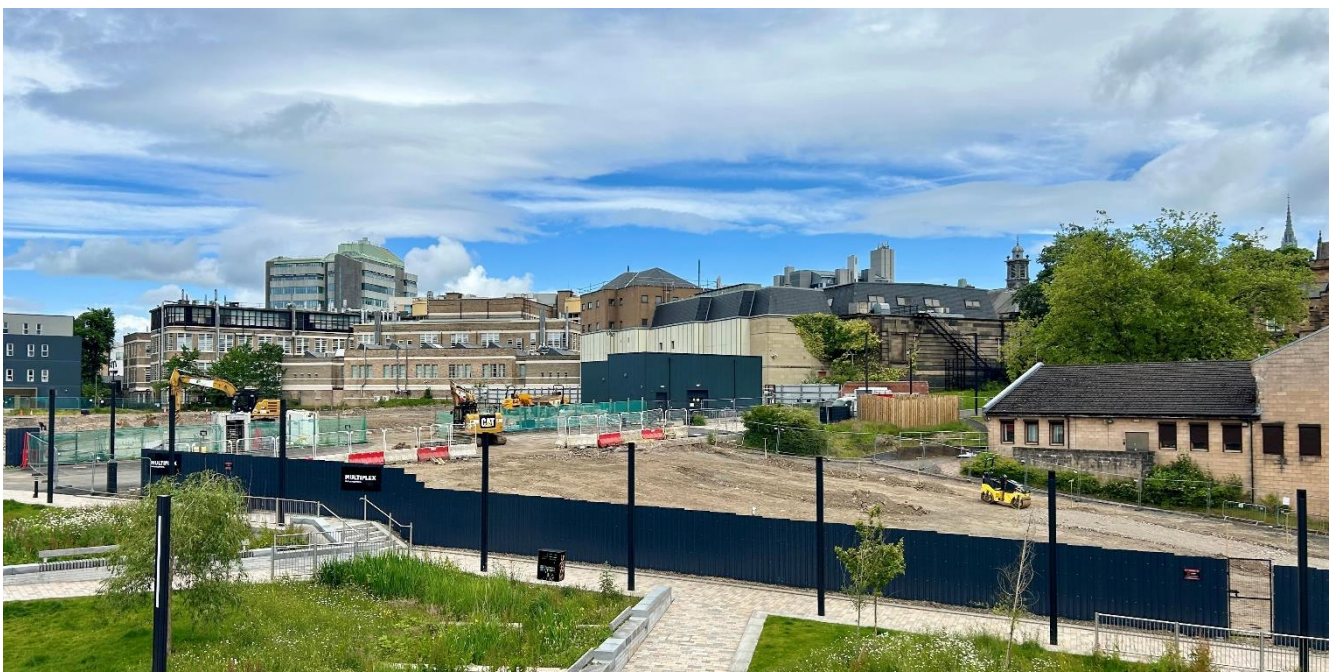
View of the enabling works from the project office
