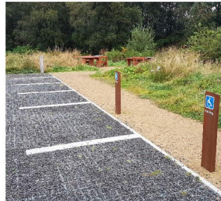
PERMEABLE CAR PARKS Forvie NNR Visitor Facilities, LUC
