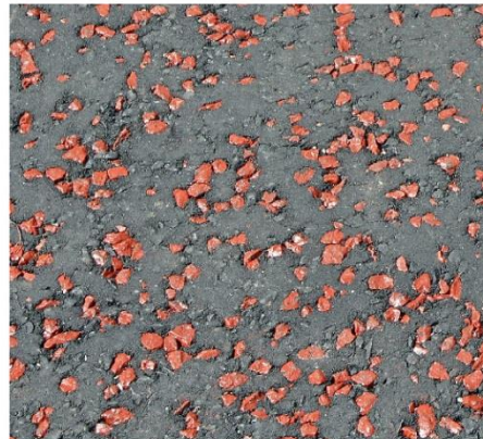
RED CHIP PAVING Cycle lane distinction
