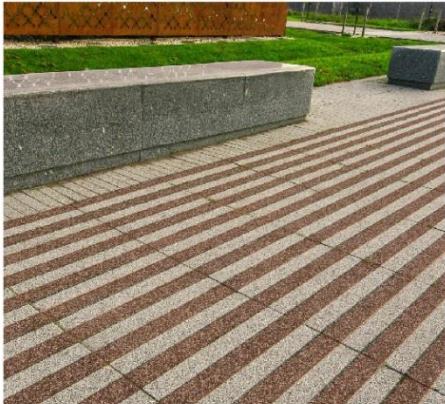
KELLEN PAVING Shawfields, LUC
